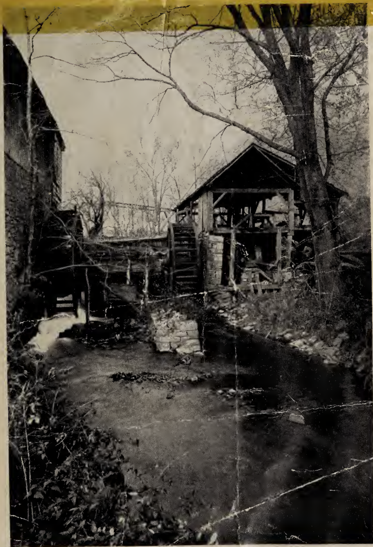
THE LAST ORNDORFF MILLS ON THE ANTIETAM
